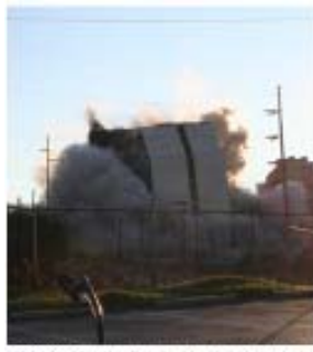
19246... Carolina Plaza tumbled down in implosion
